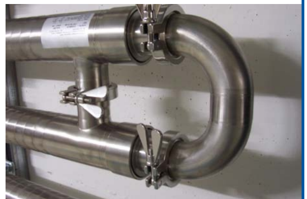
Mono-tubes with hygienic clamp connections
